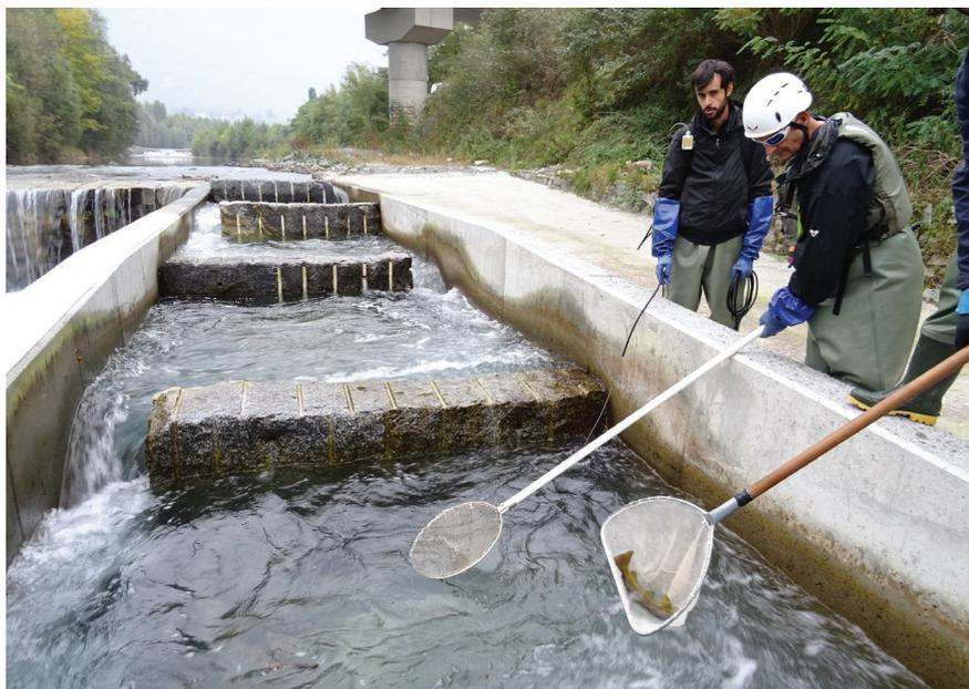
FIG.35: ELETTROPESCA NEL PASSAGGIO PER PESCI A BACINI SUCCESSIVI
